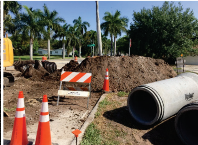
Construction storm pipe
